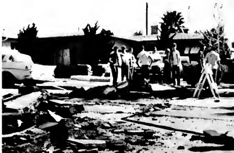
Photo 11. Day of the earthquake, looking east along thrust zone across Orange Grove Avenue, San Fernando. Wood-frame house straddles faulting in street and curbing. Note chimney, air conditioner, and TV antenna in place.
